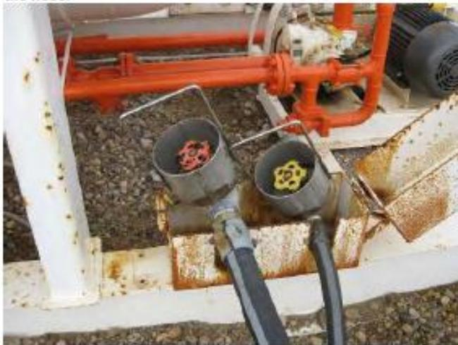
**Typical hose end valve protector. Also provides convenient way to carry the hose.**
