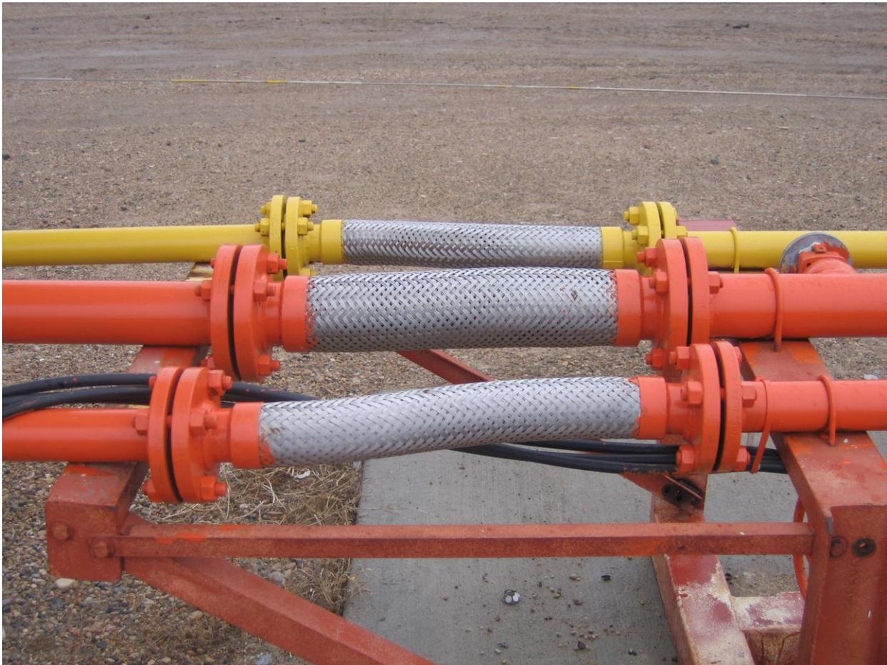
**Example of stainless steel braided flex pipe used to absorb differential movement. Flex pipe is not designed for differential movement in the axial direction, only movement at right angles to the pipe. Piping must be supported independently such that no loads are imposed on the flex pipe. Rubber hose used for this purpose must be hydrotested annually.**
