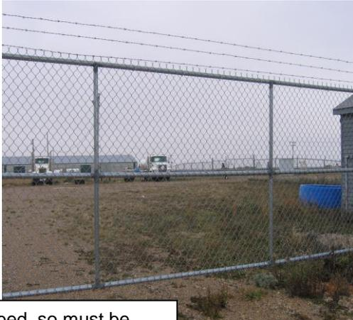
Page wire is easily climbed, so must be topped with barbed wire. Chain link fencing is preferred.
