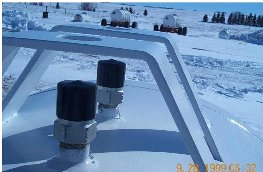
POSITIONING OF HYDROSTATIC RELIEF VALVES
