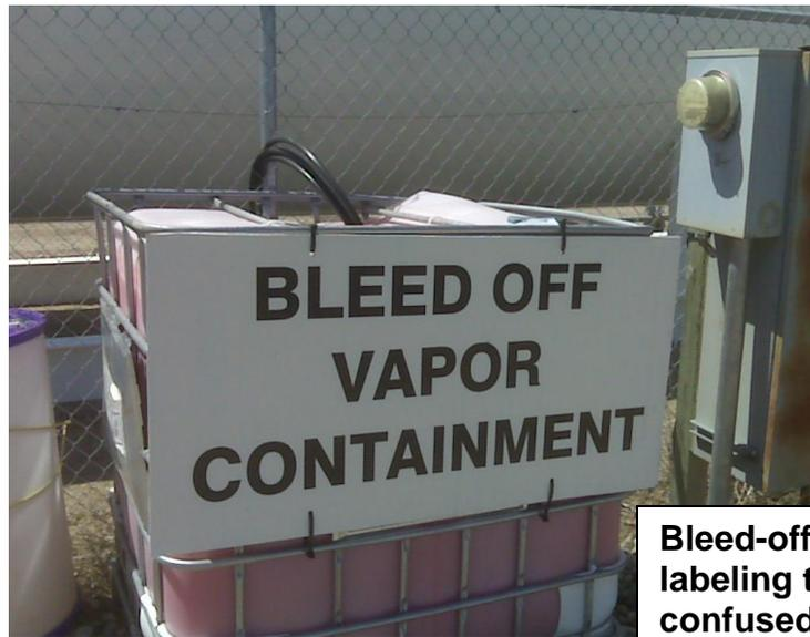
**Bleed-off tank with lid and labeling to ensure it is not confused with emergency water**
