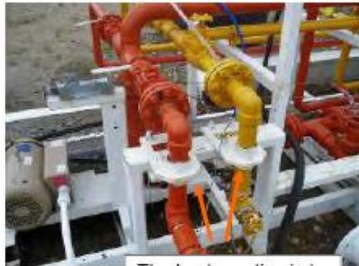
The best practice is to have piping supported to prevent damage in the event of a pull-away
