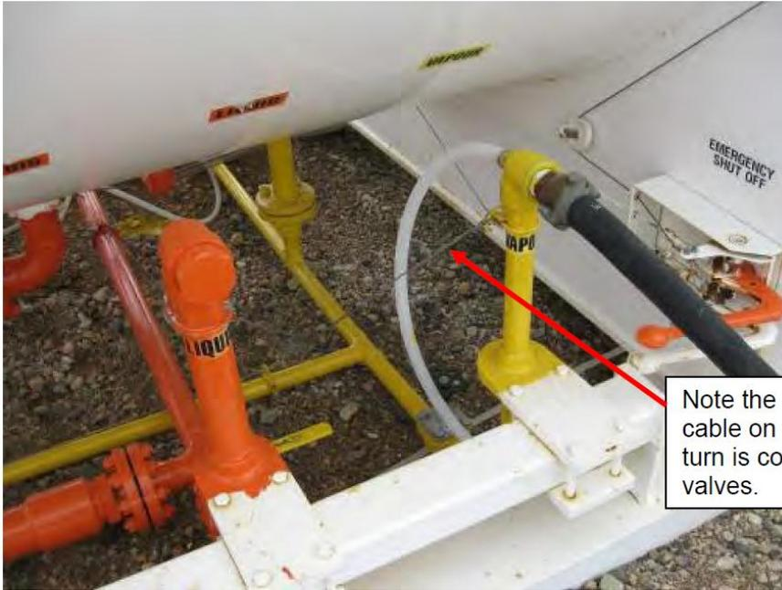
Note the pullaway protection cable on the hose riser which in turn is connected to the ISC valves.
