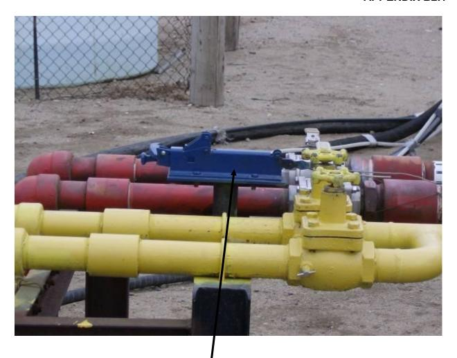
Emergency shutoff pull station (colour coded blue)
