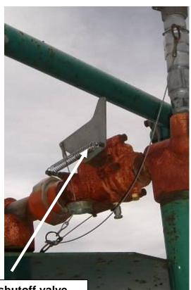
Emergency shutoff valve. Should be colour coded blue.
