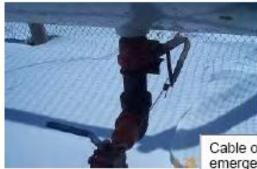
Cable operated emergency shutoff valve
