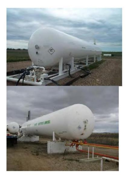
Solid, non-flammable support for the pressure vessel (and in this case, piping also).
