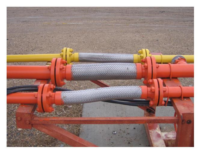
Example of stainless steel braided flex pipe used to absorb differential movement. Flex pipe is not designed for differential movement in the axial direction, only movement at right angles to the pipe. Piping must be supported independently such that no loads are imposed on the flex pipe. Rubber hose used for this purpose must be hydrotested annually.
