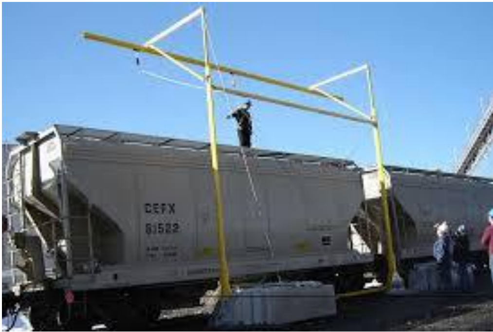
Figure 6. Example Fall Arrest with Engineered Tie-Off System
