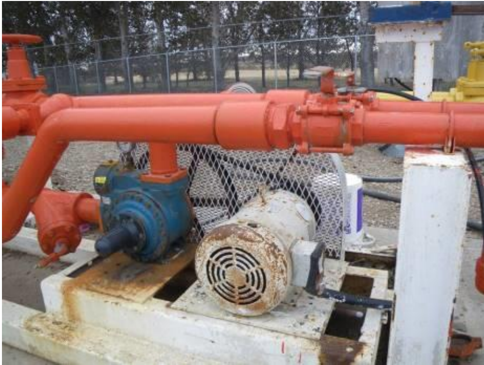
Figure 14. TRANSFER PUMP/COMPRESSOR MOUNTED
