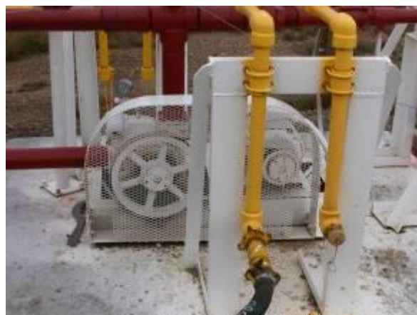
Figure 12. Guards on Transfer Pumps/Compressors – Example 1
