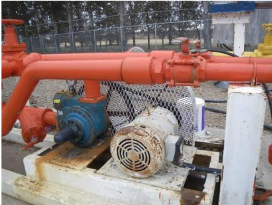
Figure 12. Guards on Transfer Pumps/Compressors – Example 1
