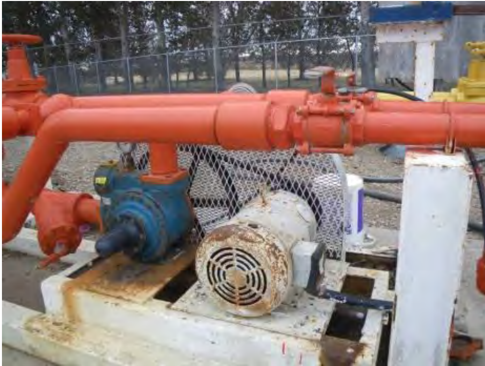
Figure 14. TRANSFER PUMP/COMPRESSOR MOUNTED
