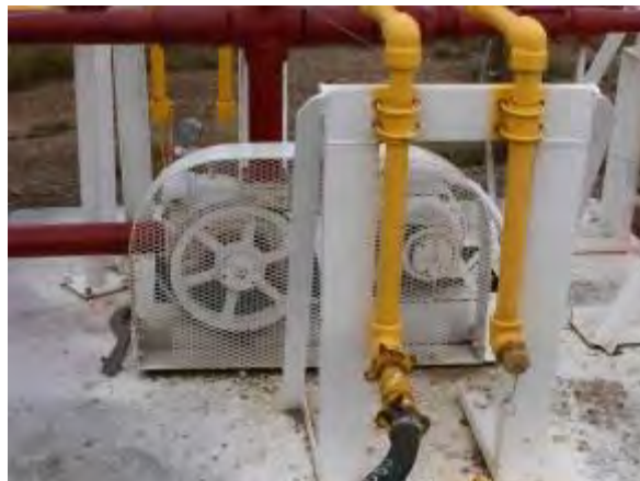
Figure 12. Guards on Transfer Pumps/Compressors – Example 1
