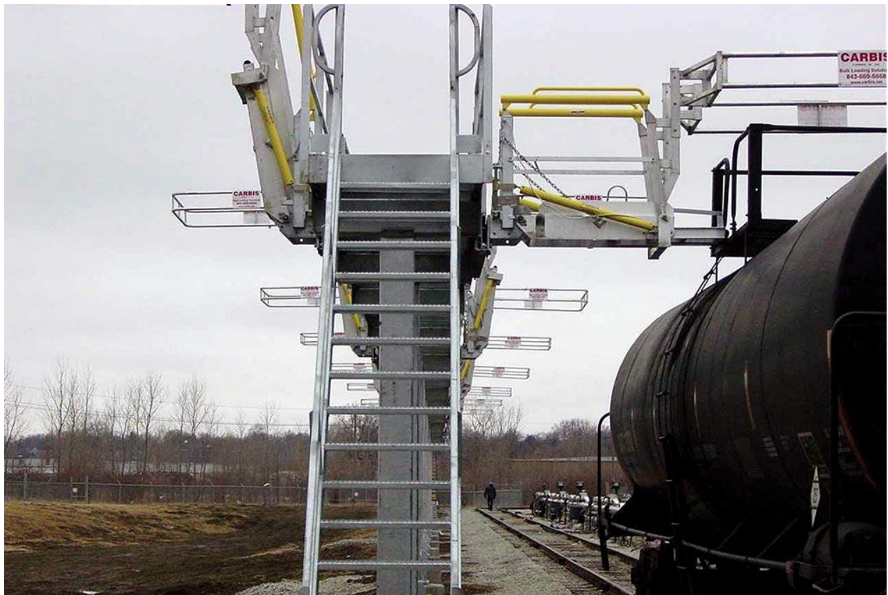
Figure 5. Example Fall Restraint System
