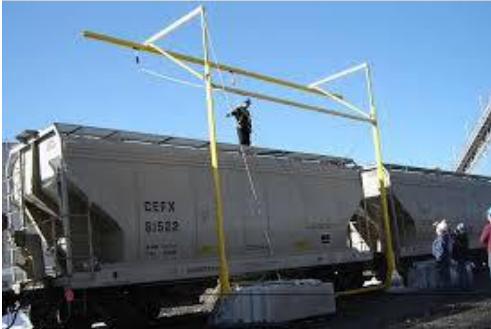
Figure 6. Example Fall Arrest with Engineered Tie-Off System
