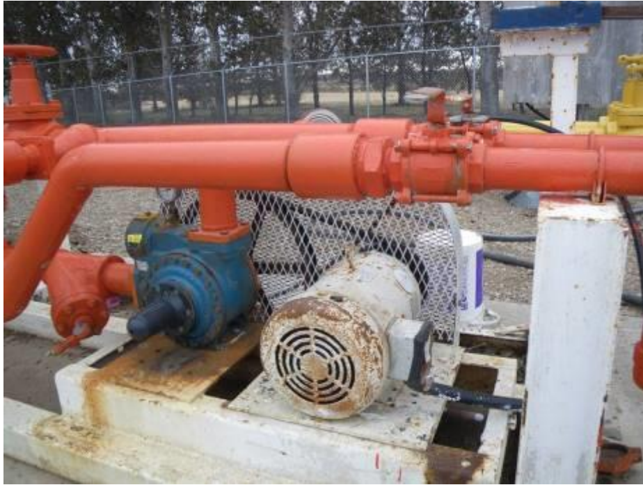
Figure 12. Guards on Transfer Pumps/Compressors – Example 1
