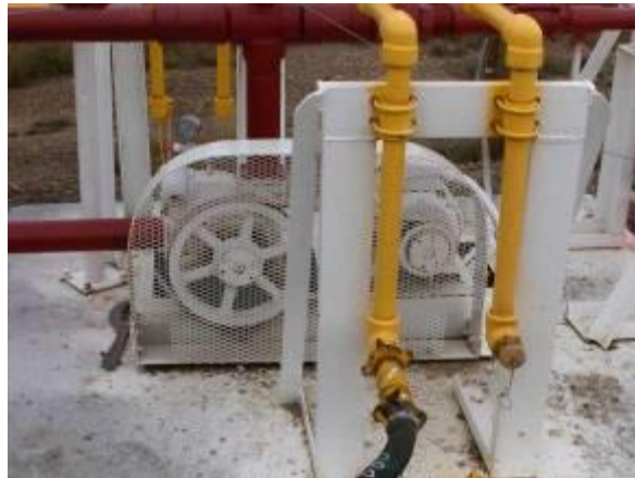
Figure 12. Guards on Transfer Pumps/Compressors – Example 1
