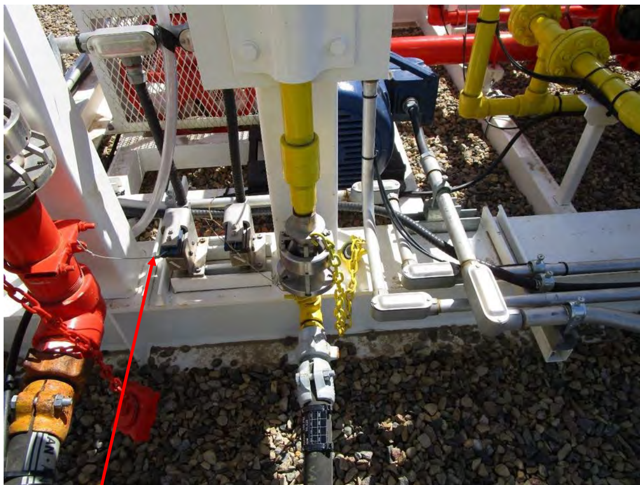
Cables connected to electronic shut down
