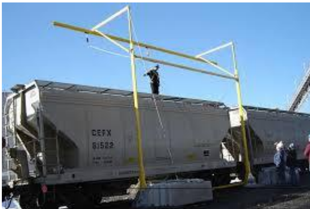
Figure 6. Example Fall Arrest with Engineered Tie-Off System
