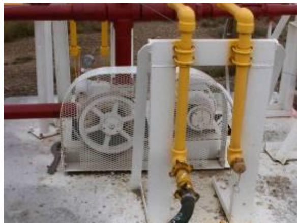
Figure 13. Guards on Transfer Pumps/Compressors – Example 2
