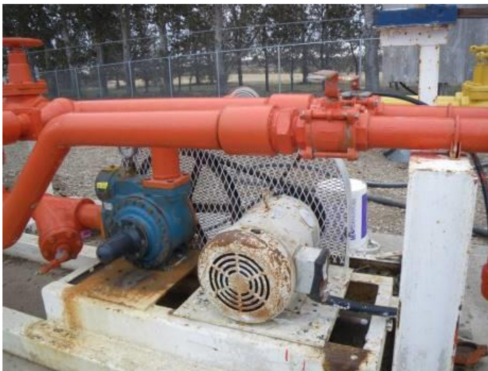
Figure 14. TRANSFER PUMP/COMPRESSOR MOUNTED
