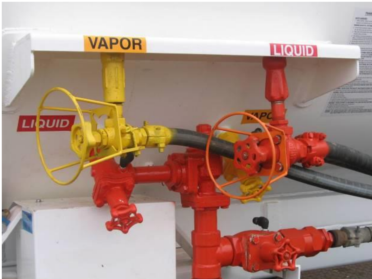
Figure 4. Typical hose end valve protectors.
