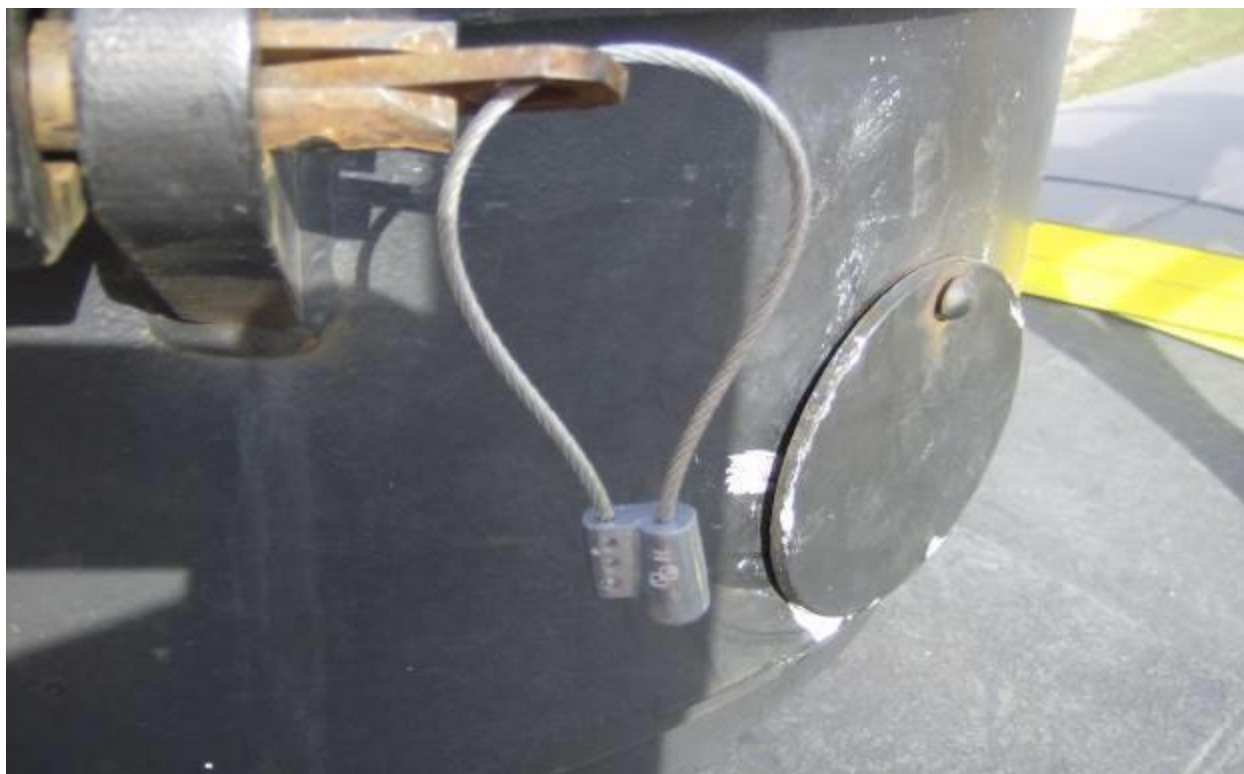
Figure 27 Cable style Car Seal
