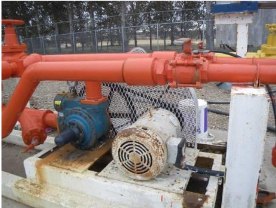
Figure 12. Guards on Transfer Pumps/Compressors – Example 1
