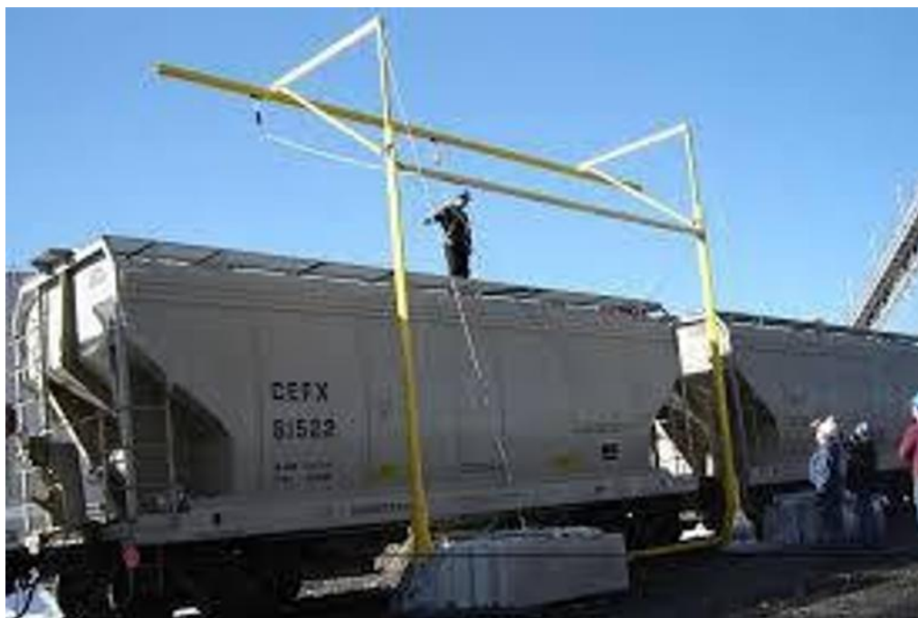
Figure 6. Example Fall Arrest with Engineered Tie-Off System
