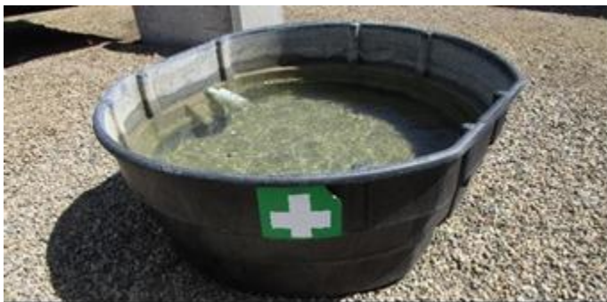
Minimum two immersion tanks (200 gallon) within 10 meters of transfer points Note that the water troughs must be marked as emergency water with white cross on a green background
