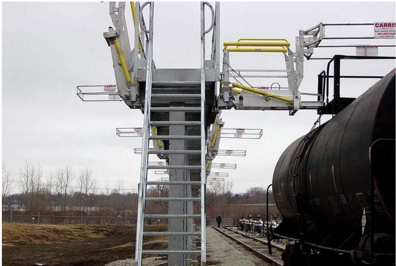
Figure 5. Example Fall Restraint System
